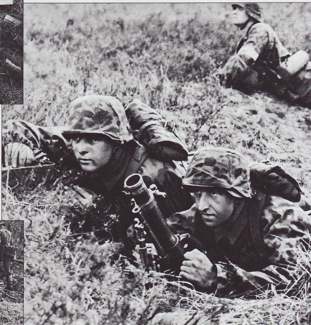
5cm le.GrW 36 mortar team take up their firing position. The le.GrW 36 intended role was to engage pockets of resistance that were beyond the range of hand grenades. The main drawbacks of the weapon were its inadequate range and the limited effectiveness of its ammunition, which were regarded as not heavy enough. (RM collection)
