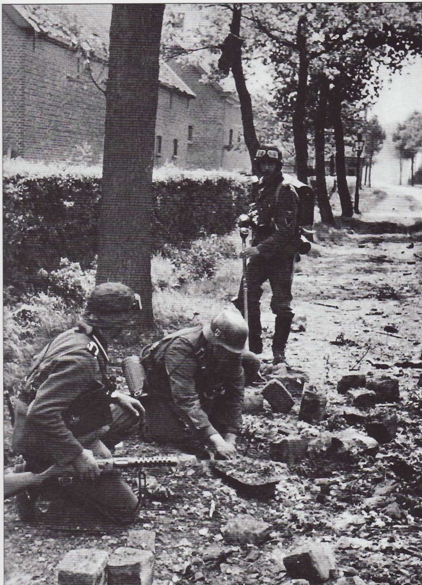
A motorcycle pioneer platoon removing mines from a road. The soldier in the background, watching the work being carried out is equipped with a knapsack mine-detector, which was still a very rare piece of equipment at the time. Note the NCO on the left armed with a 9mm 'Bergmann' MP28 machine pistol which were mainly issued to troop commanders in the field. (RM collection)
